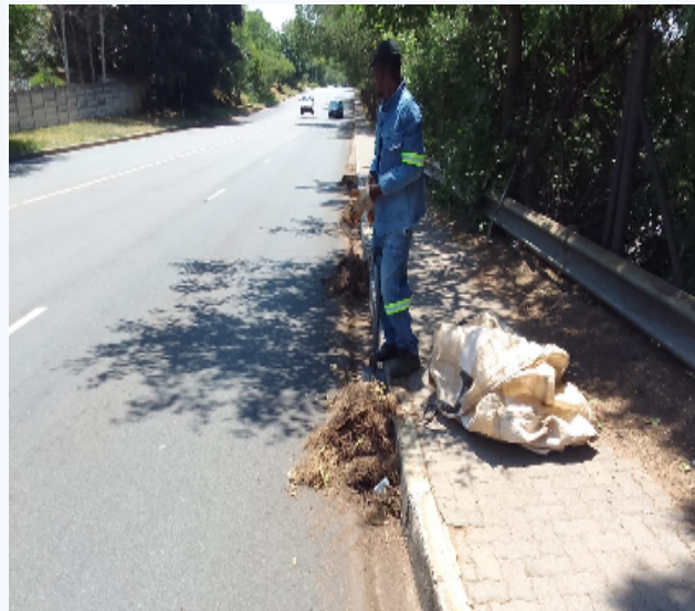
Clearing overgrown kerbs & verges
