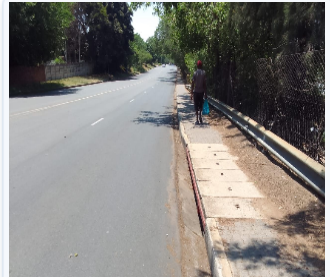
Kerbs & verges restored along the road
