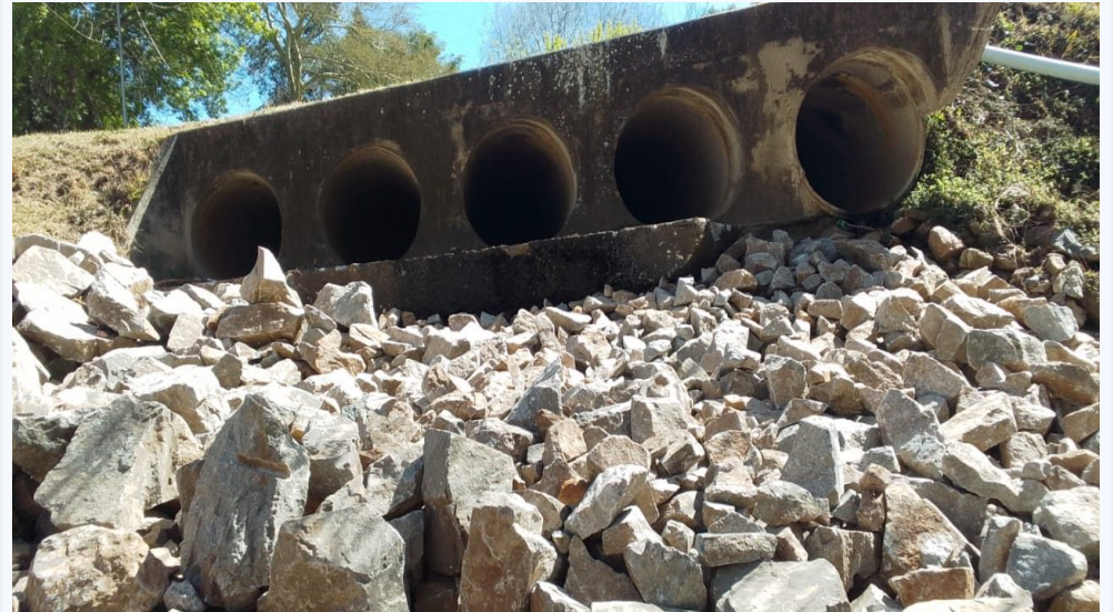
Reinforced culvert — protecting the road
