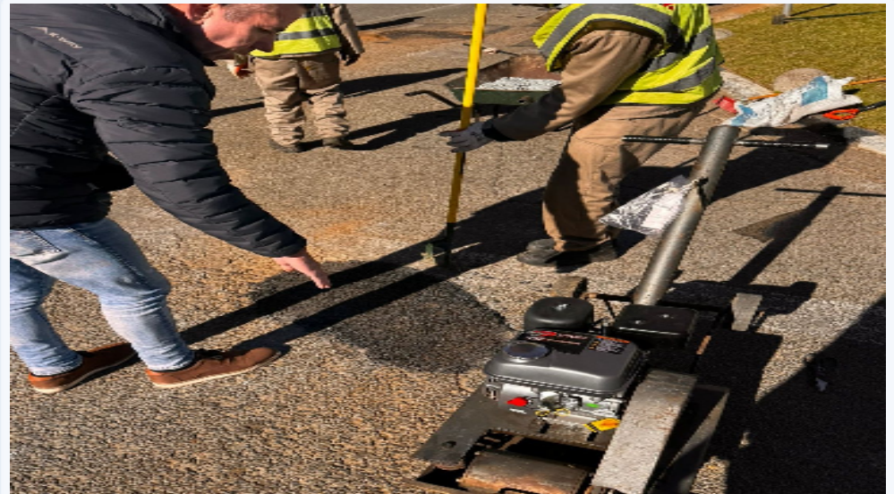
Compacting the new road surface
