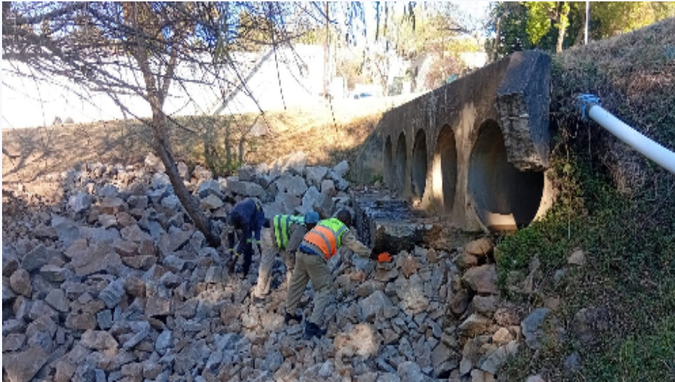
Filling the scour cavity with rock
